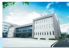
LESSO Research Institute & Testing Center
